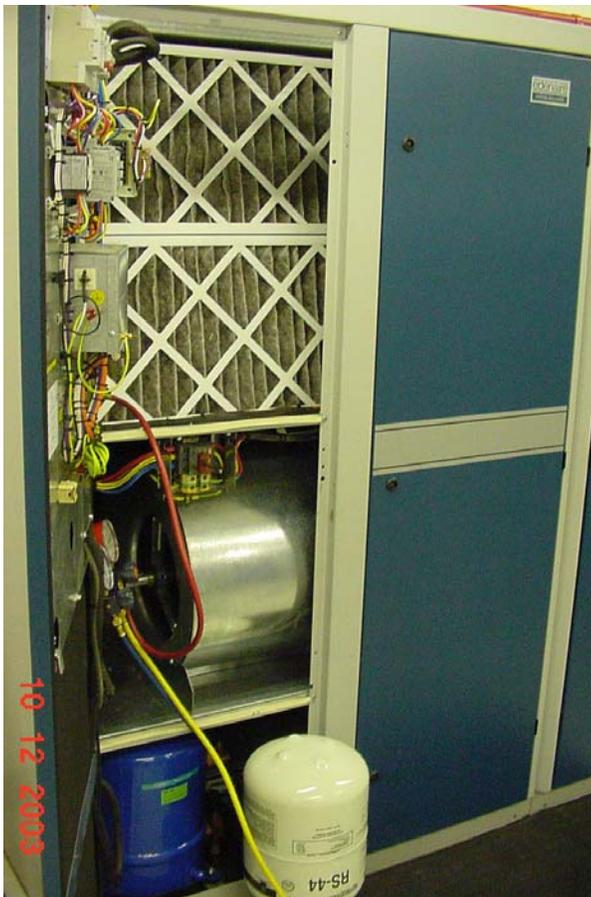
Cable and Wireless 30kW DX AHU unit being converted to RS-44 at Bristol.
