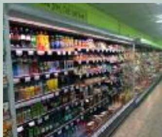
In the forefront, the new cabinet. In the background, the
